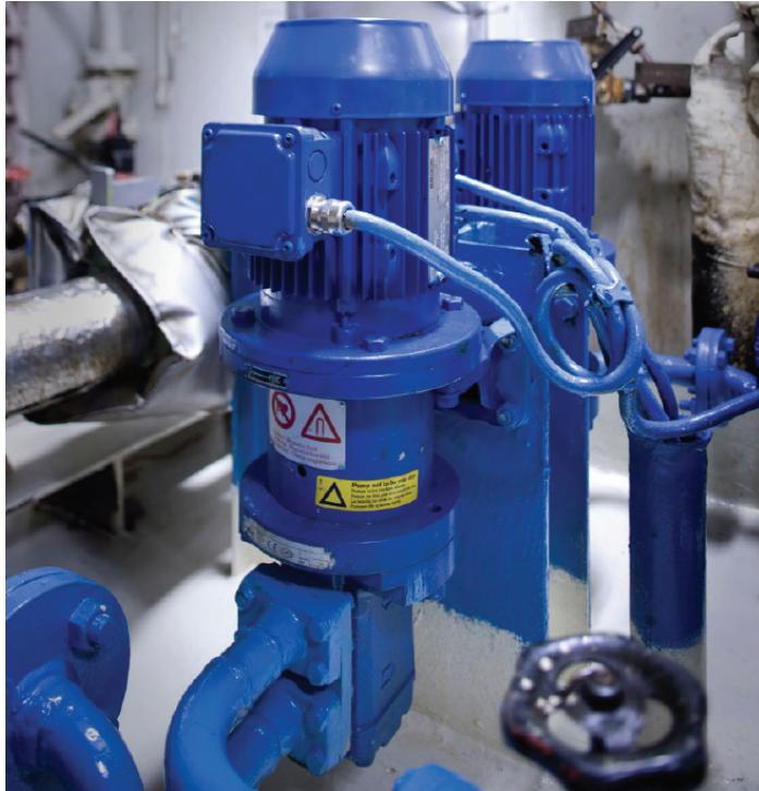
One of the world's largest tanker operators – which maintains 100 vessels and holds an International Organization for Standardization (ISO) 14001 certificate for reducing its environmental footprint – has installed 55 IMO® OptiLine pumps like this one for pumping fuel on 12 of its tankers.
